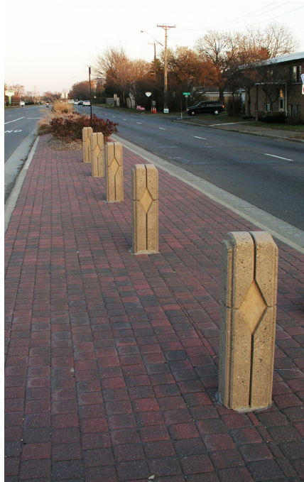
Bollards at median noses
