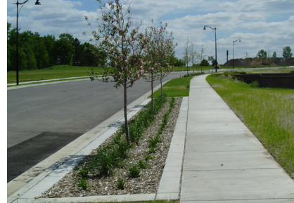
Tree trench with plantings in boulevard
