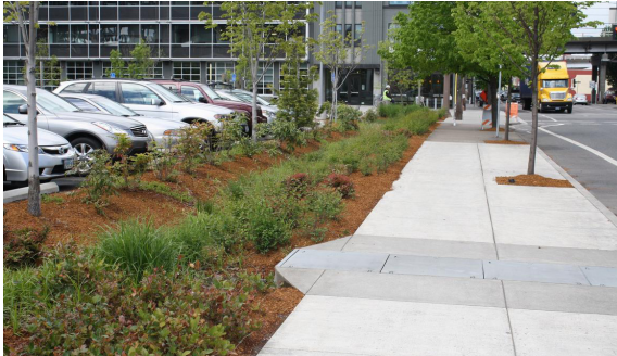
Infiltration swale along parking lot
