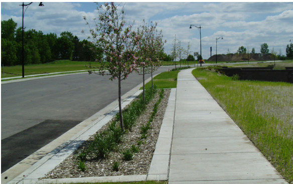
Tree trench with ornamental plantings in boulevard
