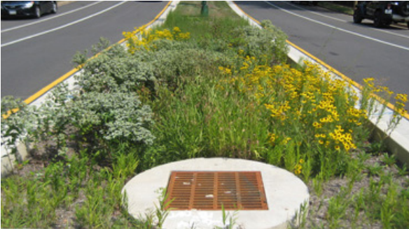
Depressed median with infiltration and plantings
