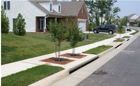
Tree trench with curb inlet in boulevard
