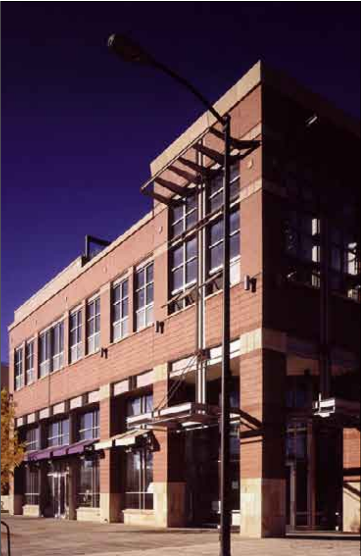
Figure 55: Details such as sills, belt courses, water table courses should be used where material transitions occur across horizontal divisions.
