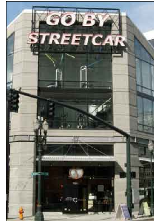
Figure 77: Screened rooftop equipment.
