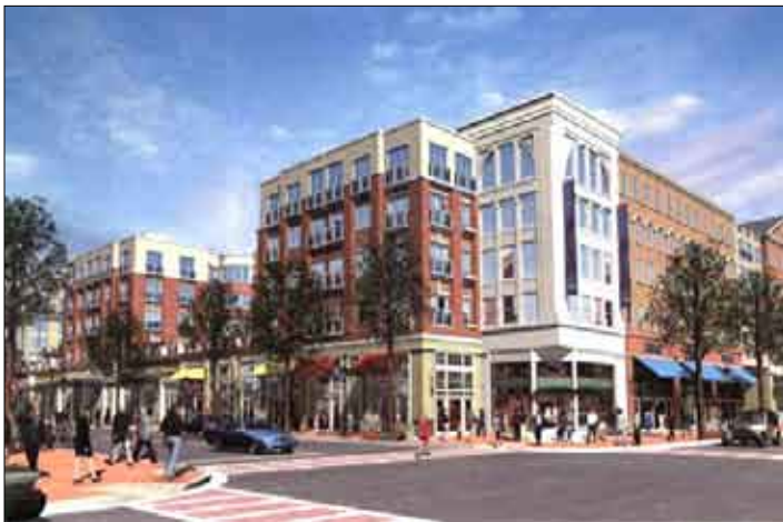
Figure 54: Use of awnings, trellis, arcades, or sign panels as elements to separate building levels are encouraged.
