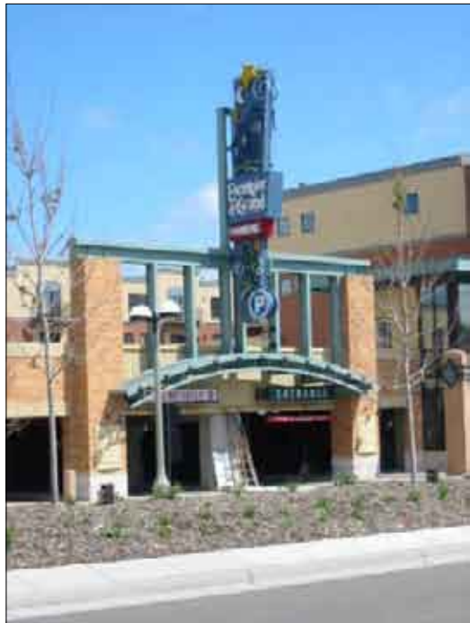
Figure 65: Detail of parking garage entrance.
