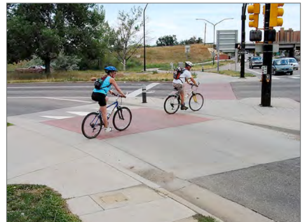
Raised and colored crosswalks reduce the speed of right-turning vehicles and improve conditions for pedestrians and bicycle riders. Image: Richard Drdul - Flickr.
