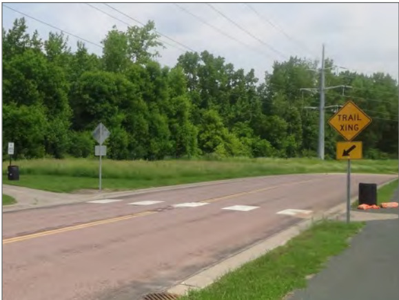
Signage and a high-visibility crosswalk help to mark this Minnesota River Bluffs LRT trail crossing along Venture Lane.
