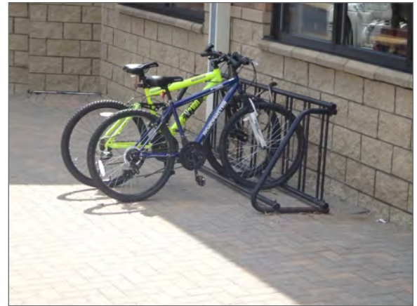
Bicycle parking currently provided at the SouthWest Station. This style of rack does not secure a bicycle’s frame, and does not provide stable parking. “Inverted-U” bicycle parking is recommended instead.
