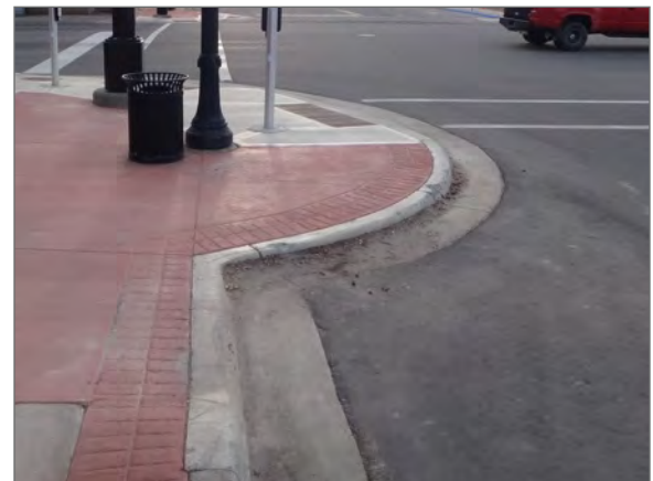
A curb extension (in Grand Rapids, MN) reduces the distance a pedestrian has to travel when crossing the road.
