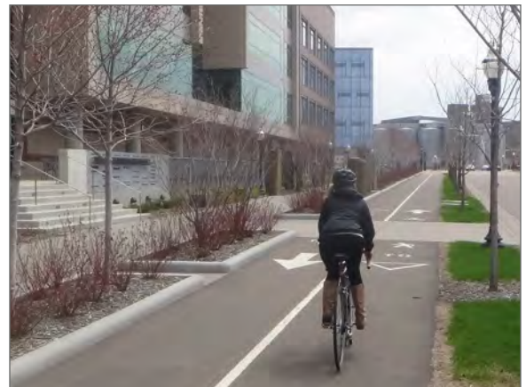
This University of Minnesota cycletrack offers physical separation from motor vehicles (on the right), and from pedestrian circulation and building entrances (on the left).
