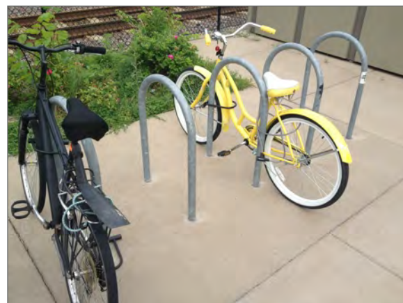
Inverted-U style bicycle parking should be installed near the primary entrances to buildings.
