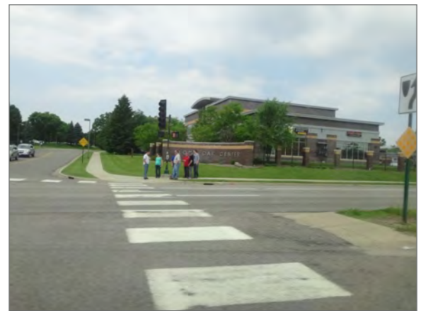
Pedestrians waiting to cross Mitchell Road at Lone Oak Road in Eden Prairie. This intersection has a good high-visibility crosswalk, but would benefit from a “bull-nose” extension of the median beyond the crosswalk to create a refuge island, as illustrated on the next page.
