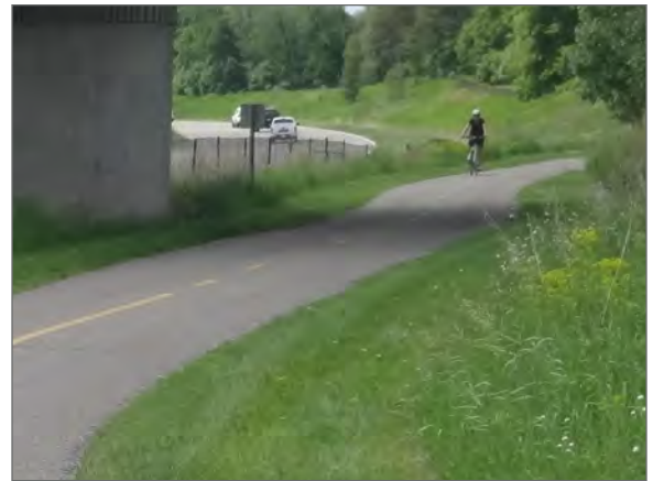
The Minnesota River Bluffs LRT Regional Trail provides regional connections between Eden Prairie and surrounding communities.
