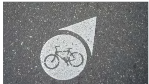
“Route dots” marked on the pavement can be used to offer route guidance in residential areas. In the case shown, the route veers to the right.
