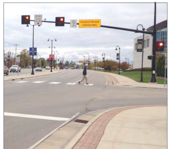
Pedestrian Hybrid Beacon (PHB, or HAWK) at a crossing of Division Street in St. Cloud.
