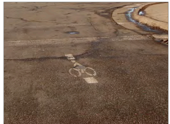
A pavement marking to help bicycle riders to position to activate a traffic signal to cross.
