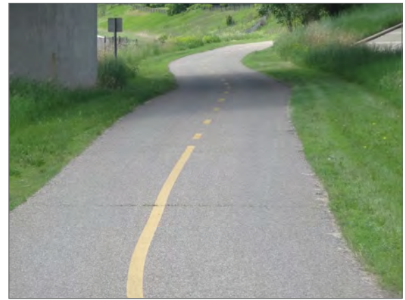
The center line changes from solid to dashed, indicating it is safe to pass.
