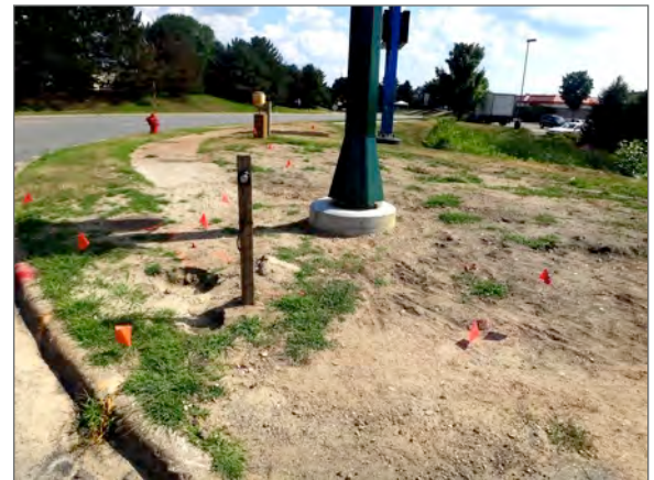
Construction work in Eden Prairie.
