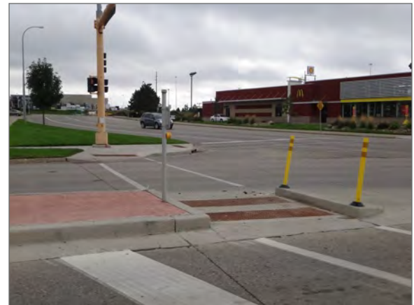
A “bull-nose” refuge island extends the median beyond the crosswalk and provides additional protection to pedestrians.
