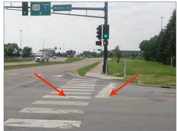
A continental crosswalk and vehicle stop bar at Martin Drive and Mitchell Road in Eden Prairie.
