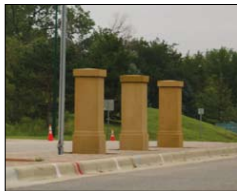
New bollards lining Technology Drive.
